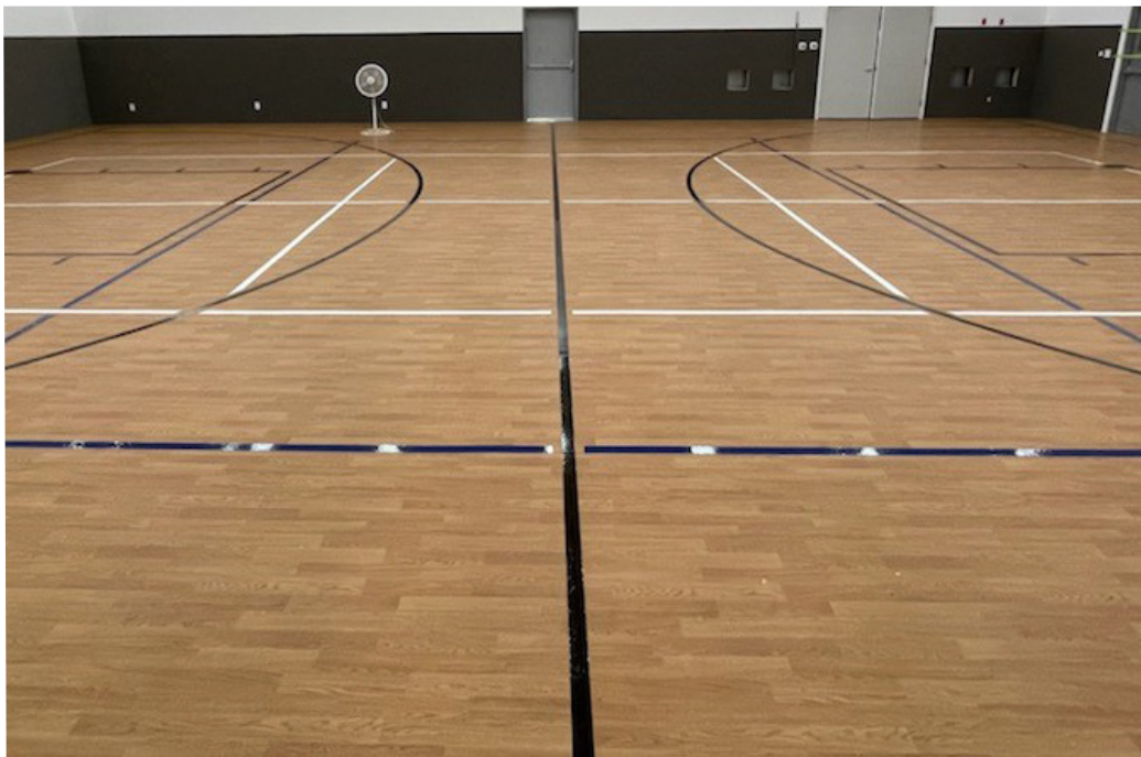
Installation prior to game lines application
